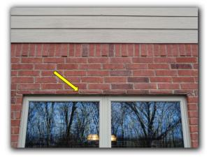
One or more hairline cracks at brick/mortar. Indicative of general settlement, not excessive at time of inspection.
