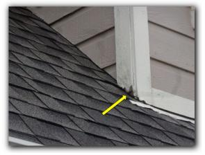
Open caulk joints at one or more locations-(doors, windows, and/or trim boards) at the exterior of the home. This is considered a routine maintenance issue and will need to be re-sealed periodically. Location examples: trim/siding junctions, exterior wall entry points(AC cutoff, electric meter base, AC refrigerant line)
