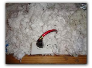
Note: plugs in the home are not tamper resistant type. Per today's building standards all plugs 5.5 ft above or closer to the floor should be. Common for home this age not to have tamper resistant type. This is for child safety. After market safety devices can be installed for safety.
