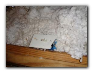
Note: extension cord plugged into receptacle near attic access, unsure what this is supplying power to, suggest ask seller.
